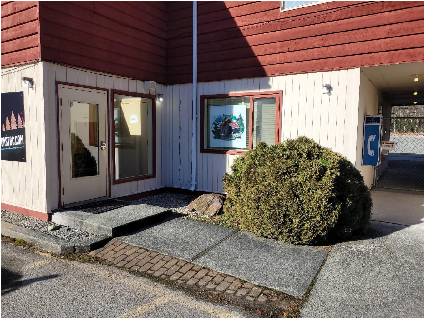
Terminal – South East Entrance to Stairwell
