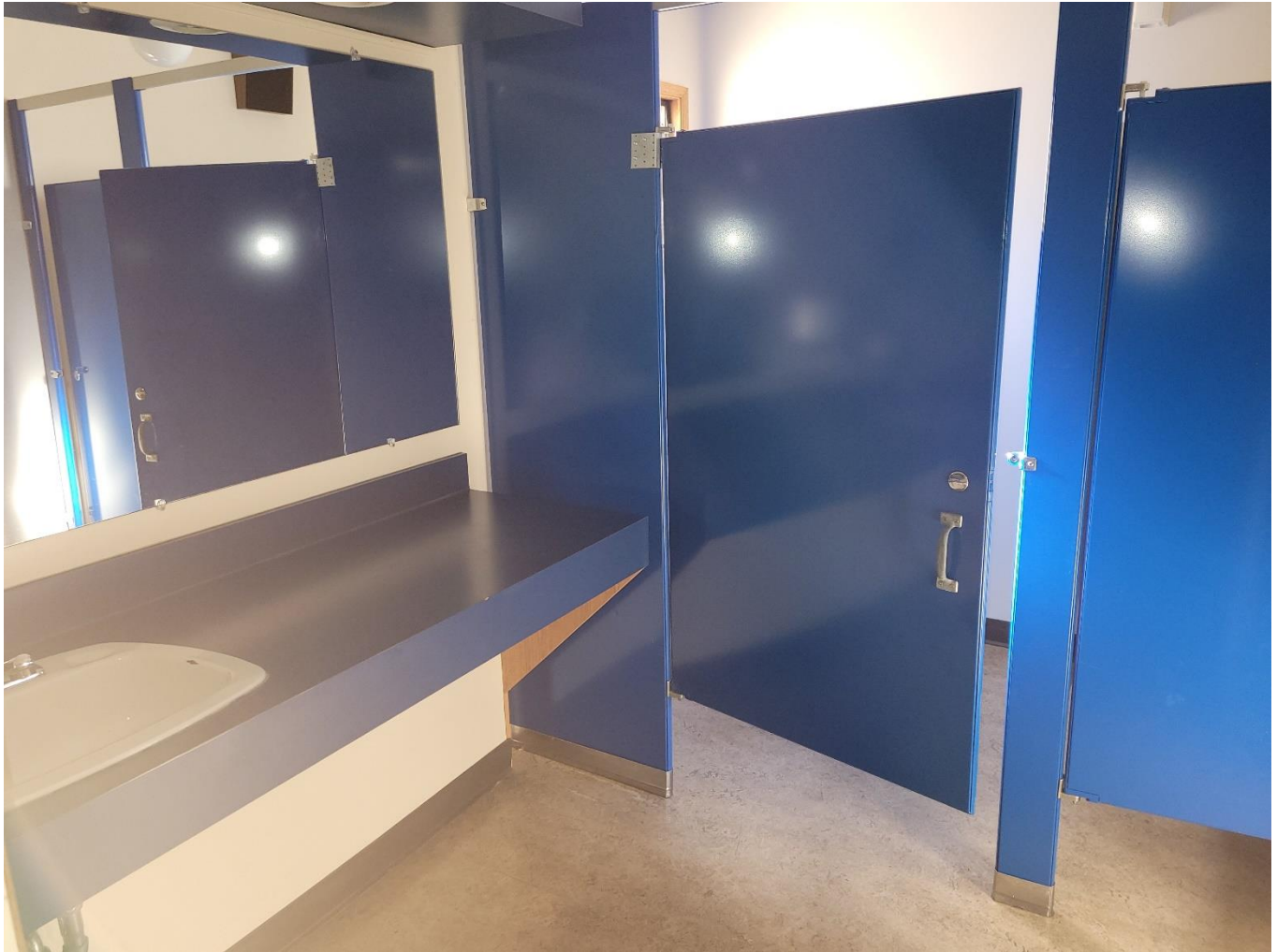
Terminal – Ladies Restroom
