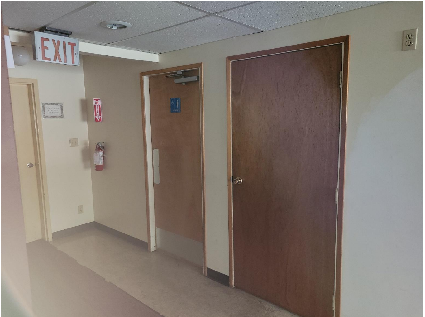
Terminal – Ladies Restroom and Storage Room
