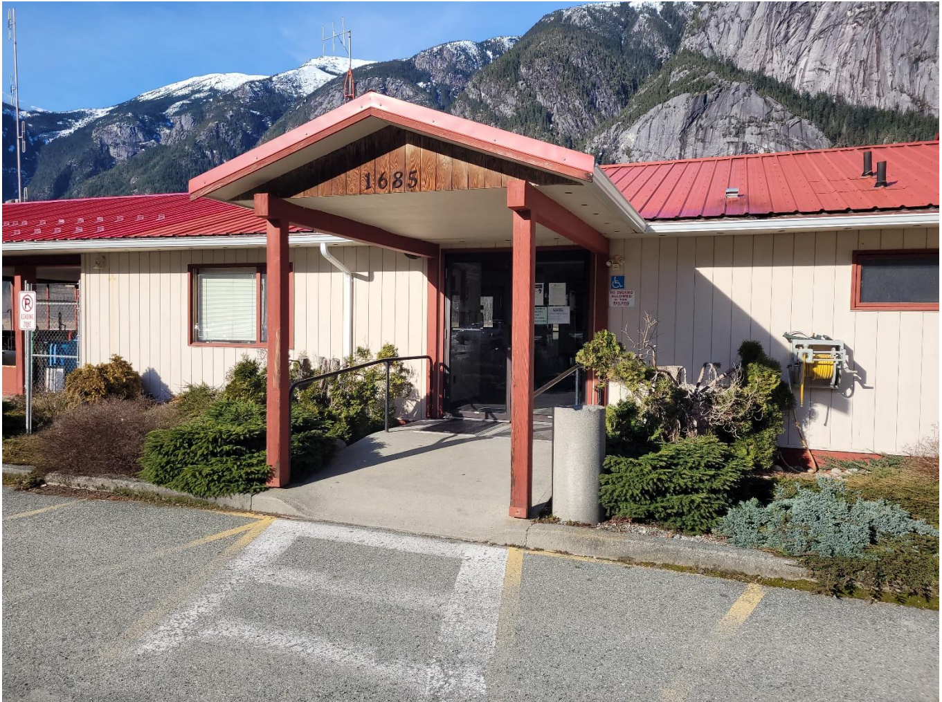
Terminal - Existing Front Entrance
