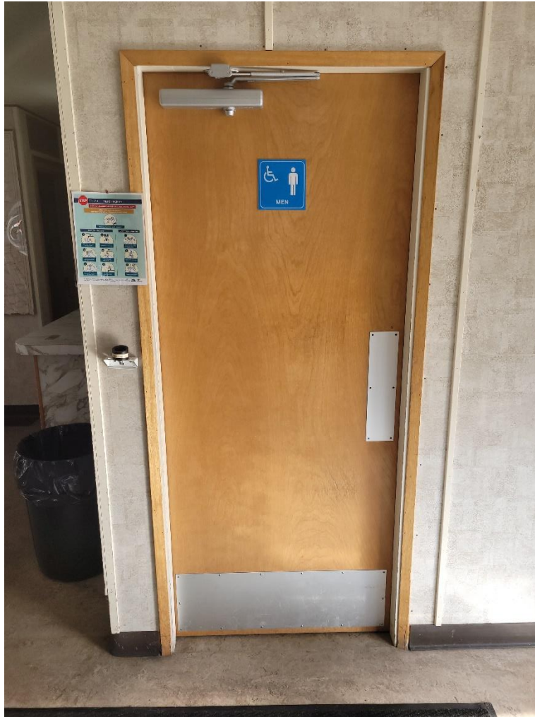
Terminal – Men's Restroom Entrance
