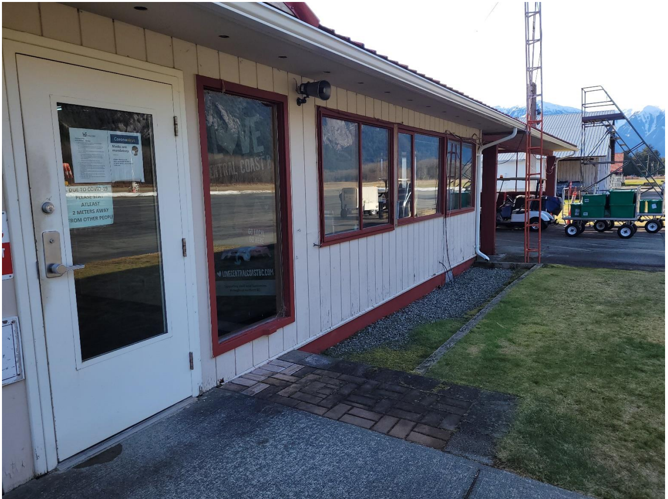
Terminal – South Airside Entrance
